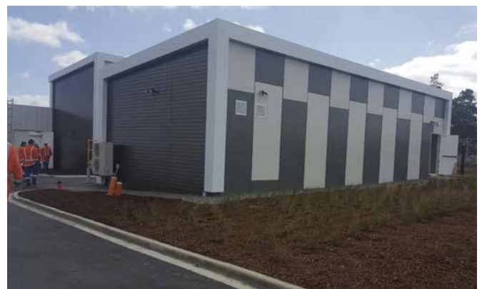
Above: the completed switchroom and transformer buildings on site. Images supplied by Connell Contractors.
