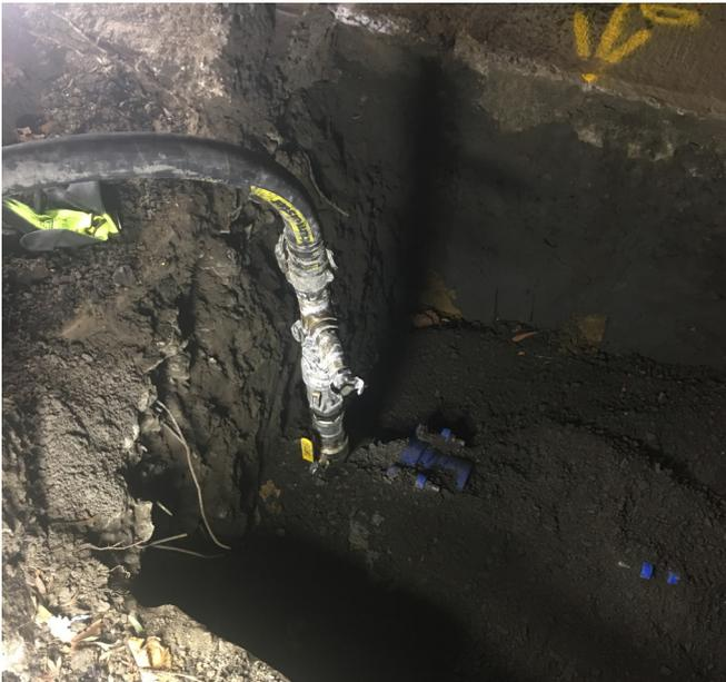
Gas main pipe to be filled with Terefil®
