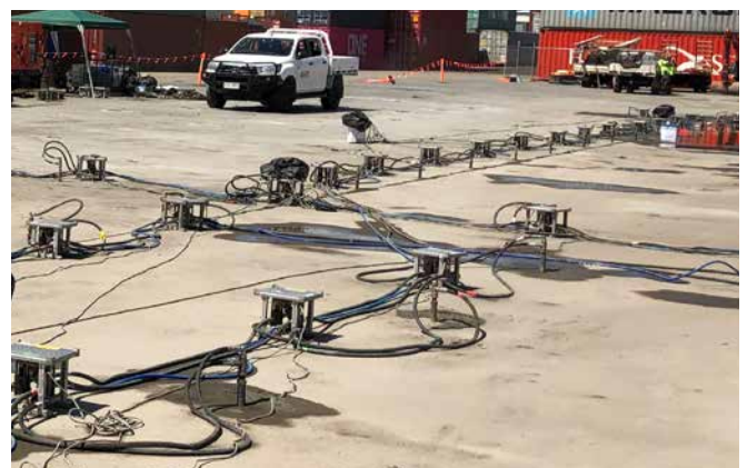
Mainmark installed a total of 400 JOG injection points.
