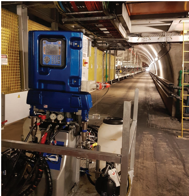
Mainmark's customised rig
