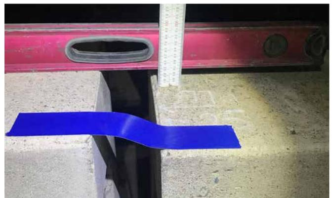
The Mall bridges' subsidence was most clearly seen in the variation of levels on the pedestrian walkway walls.
