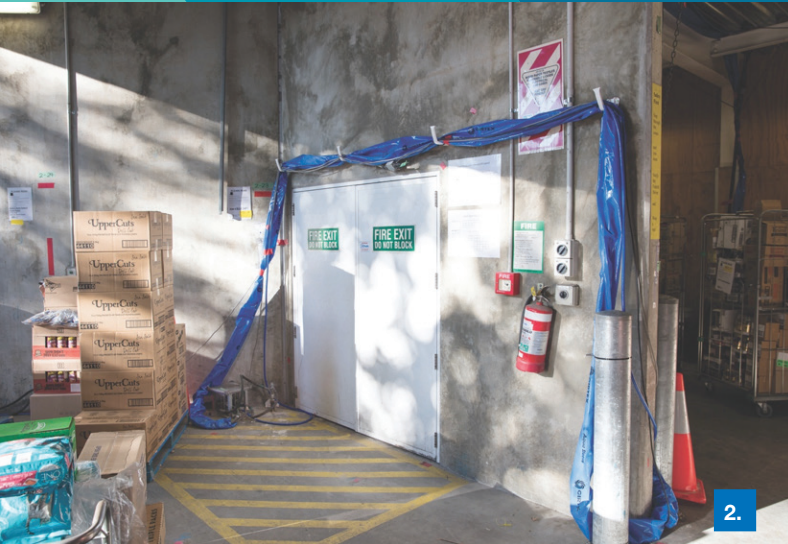
2. Customised installation of required hoses and cables allowed tenants to remain fully operational during the project without compromising health and safety. 3. Internal injection works carried out at night; full store operations restored by opening everyday.
