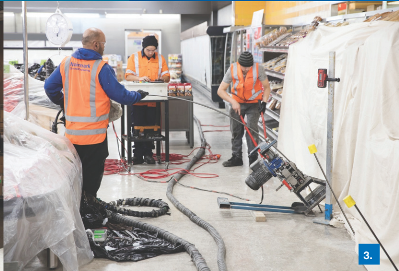
2. Customised installation of required hoses and cables allowed tenants to remain fully operational during the project without compromising health and safety. 3. Internal injection works carried out at night; full store operations restored by opening everyday.
