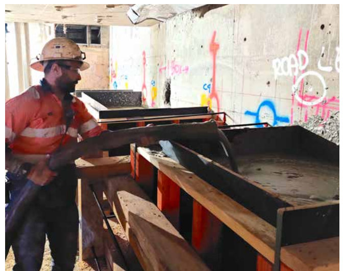
Terefil® being poured to pre-fill pile form
