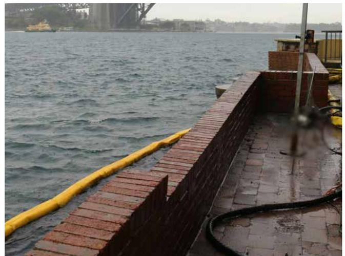
Filling the voids behind the sandstone blocks, re-supporting the seawall, and lifting and re-levelling the patio area
