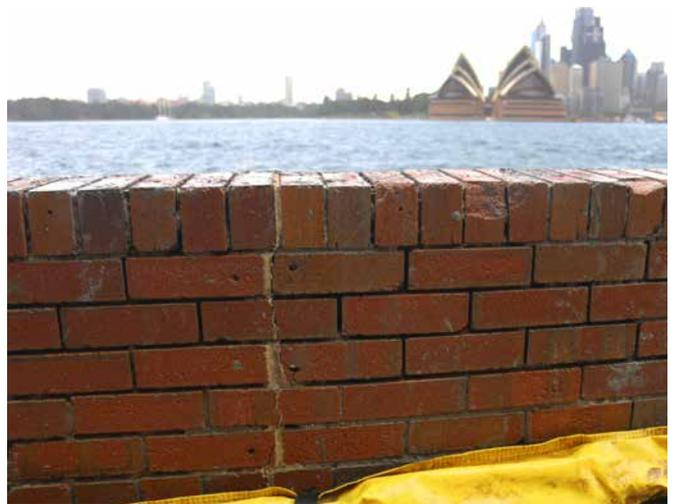
Cracks in sea wall of the property due to continuous water movement, subsidence and erosion
