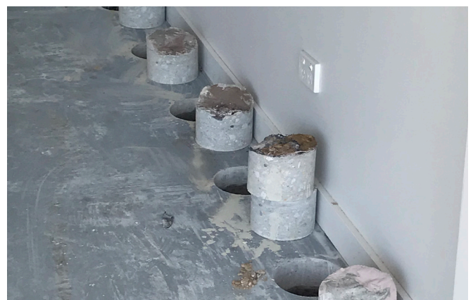
Holes prepared for injection of permeation grouting
