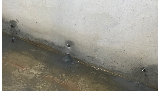
Injection points across basement walls
