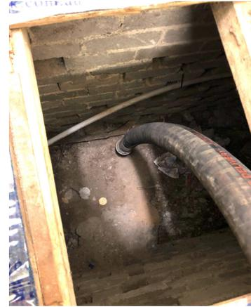
Terefil being pumped in contaminated subfloor of building
