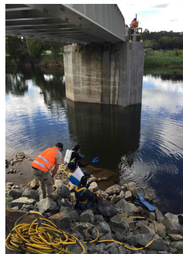
Divers preparing to inspect scour
