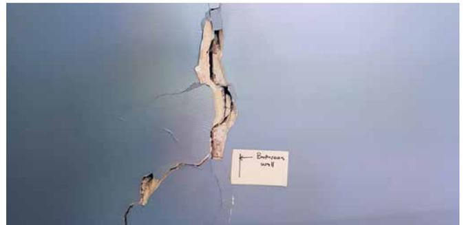
Before injection of Teretek engineered resin
