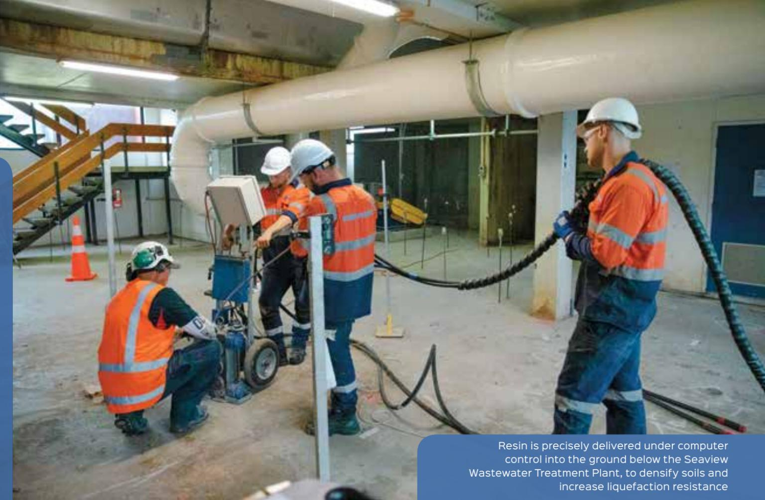
Resin is precisely delivered under computer control into the ground below the Seaview Wastewater Treatment Plant, to densify soils and increase liquefaction resistance
