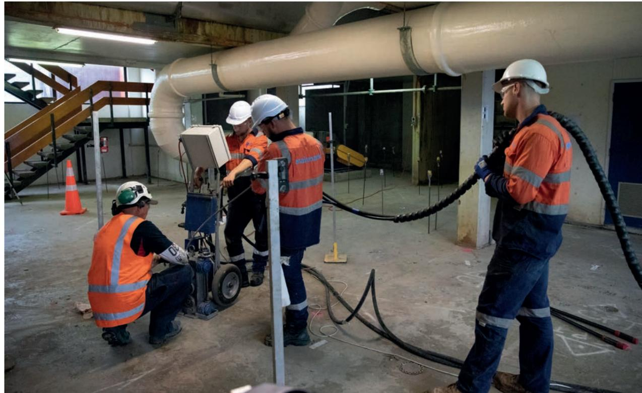
Resin being precisely delivered under computer control, according to engineered specifications.
