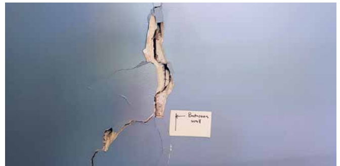
Before injection of Teretek engineered resin
