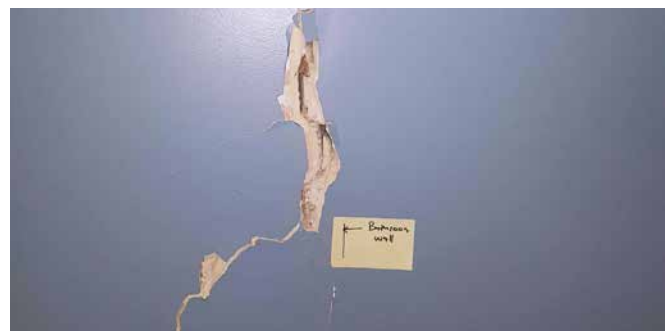
After injection - ready for final patching and painting.
