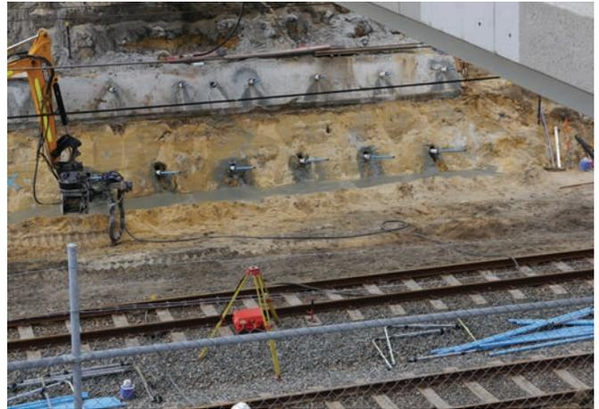
Installation of 9m deep Hollow Bar Soil Nails
