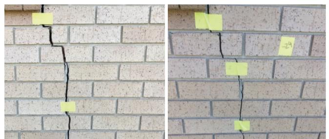
Before and after Teretek® engineered resin being injected
