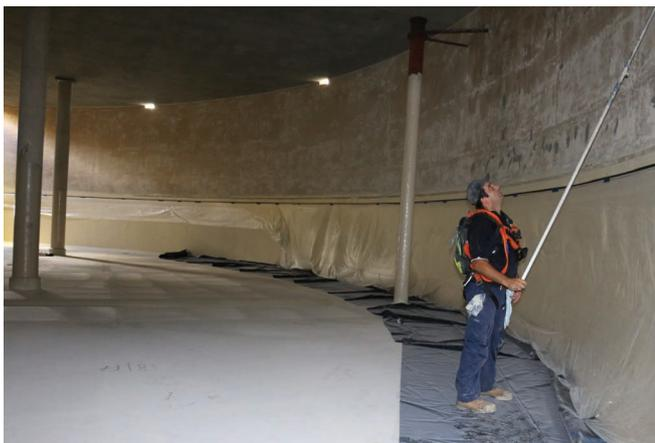
Mainmark technician applying polyurea product on the wall of the water tank
